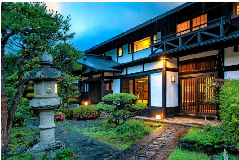
Built in 1819 and Registered as a tangible cultural property by the Agency for Cultural Affairs
